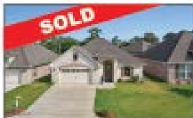
217 PARKWAY VILLAS CIRCLE DIAMONDHEAD
